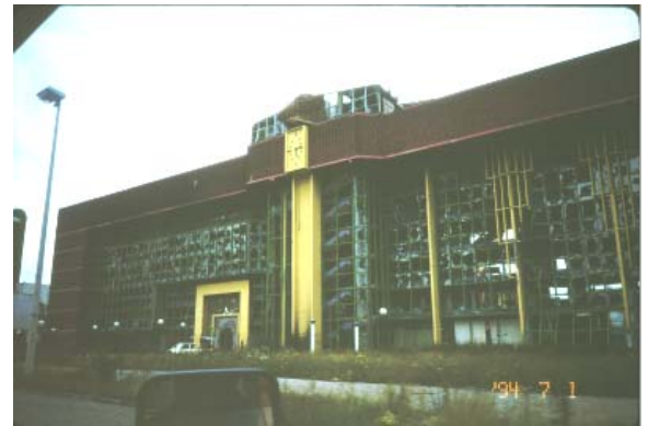
Heavily damaged building in Sarajevo
