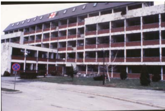
Hospital in ruins
