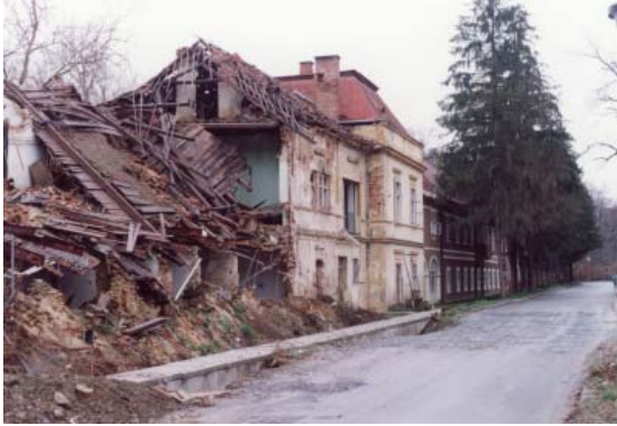
Daruvar, Croatia - damaged building next to hotel
